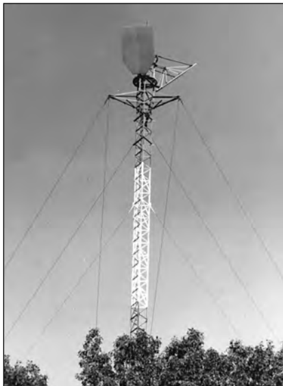
Figure 15.114 — Commercial periscope antennas, such as this one, are often used for point-to-point communication.
