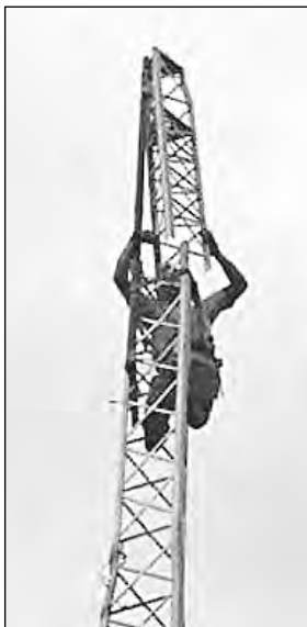
Figure 26.30 — Tower worker lowering a new section onto the top of the assembled stack of sections. The gin pole attached to the left leg is bearing the weight as the tower worker gives verbal instructions to the ground crew pulling on the haul rope. (Mike Hammer, N2VR, photo)
