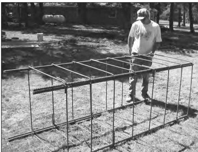
Figure 26.34 — The rebar cage for KX8D's tower base. (Duane Durflinger, KX8D, photo)
