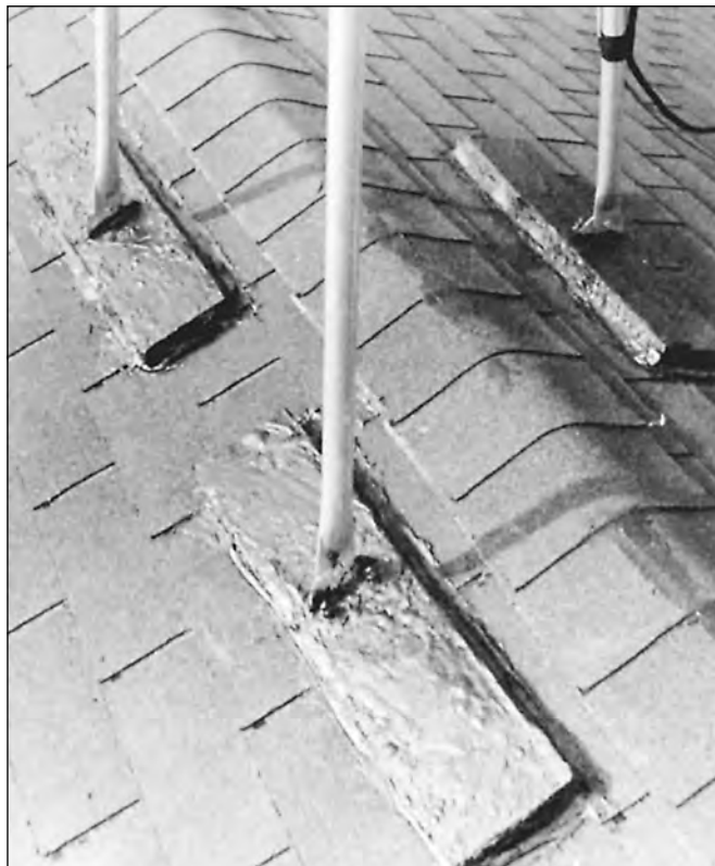
Figure 26.16 — Lengths of 2 × 6 on the roof act as footing for the tower legs and are coated by roofing tar to protect against weathering and prevent leaks. (Photo by Jane Wolfert)
