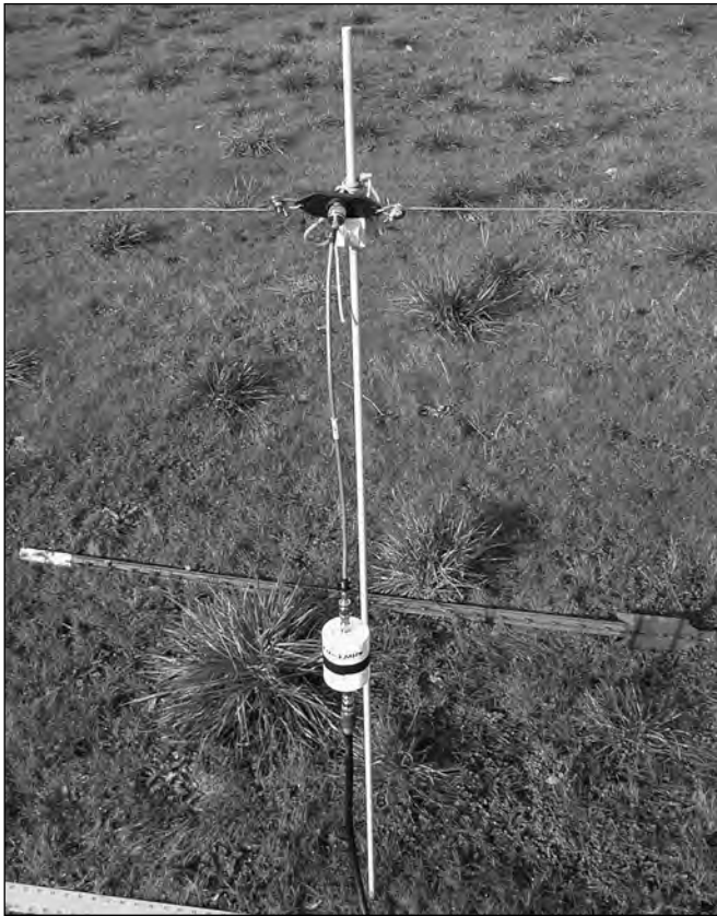
Figure 3.63 — Center connector and feed point support. Note use of a common mode choke at the feed point to isolate the feed line shield.
