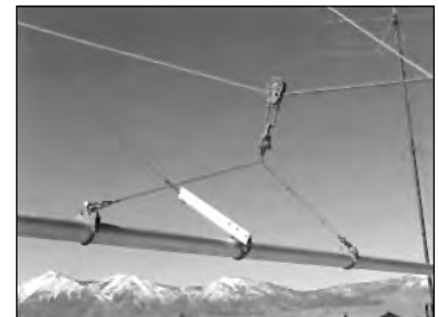
Figure 26.45 — Photo of the tram suspension system used by K7NV. Note that the tiller is attached to the haul rope in this system. The boom of the antenna can be rotated in the U-bolt holding it to the tiller to adjust the tilt of the elements to clear guy wires. (Kurt Andress, K7NV, photo)
