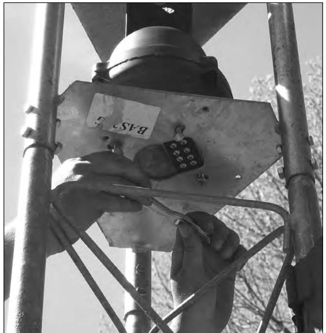
Figure 26.51 — The accessory shelf in a Rohn 25G top section is pre-drilled with a standard bolt layout to fit the popular Ham-M/1/2/3/4/V series of rotator base plates. This rotator uses a terminal strip for connections although rotators are available with waterproof connectors. After-market kits for converting rotators with terminal strips to waterproof connectors are also available.
